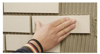
**3.** The thin bricks must be pushed into the fresh mortar bed before skin formation occurs. A beginning skin formation on the mortar on the wall reduces the adhesive qualities. This always occurs if the mortar is applied to the wall too early.
