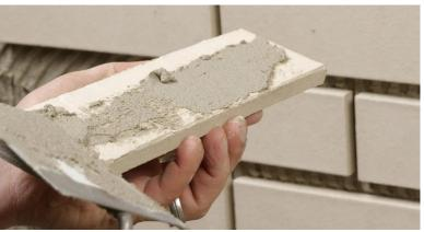
**2.** Only the combined laying method (floating / buttering method) should be used for the attachment of thin bricks, in which both the surface and the back of the thin bricks are covered smoothly with the adhesive. These results give a significant increase in the achievable adhesive tensile strength compared to the floating method.
