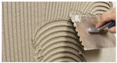
1. The mortar is applied to the setting surface in two work steps. In the first step, a smoothing trowel is used to apply a thin layer of adhesive mortar to the surface. In the second step, the layer thickness required for combing is applied to the fresh layer. The mortar layer thus produced is combed with a comb trowel, at an angle of approx. 50 angle.
